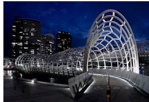
Webb Bridge (2003) Robert Owen and Denton Corker Marshall
